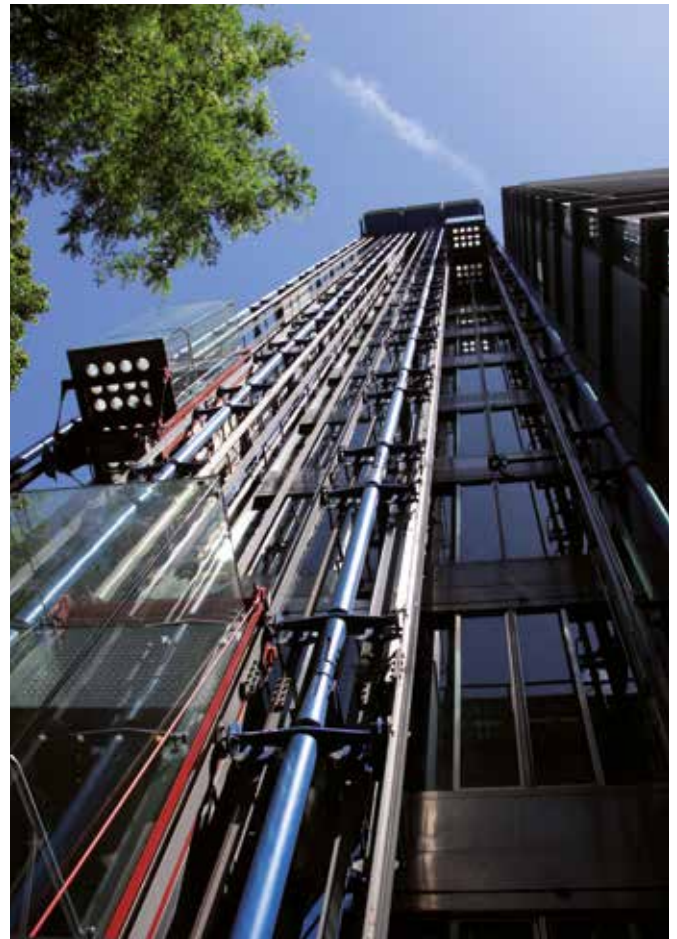
The two front towers each have four external wall climbing lifts; seen here is a bank of three lifts on one side of a tower. The glass-walled lifts offer spectacular views across London.
