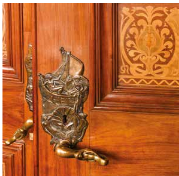
The mahogany entrance doors have handles shaped as dolphins and sea sprites and escutcheons with mermaids and sprites, all in patinated bronze. The doors have the same rosewood and fruitwood inlaid decoration as the dado around the room.
