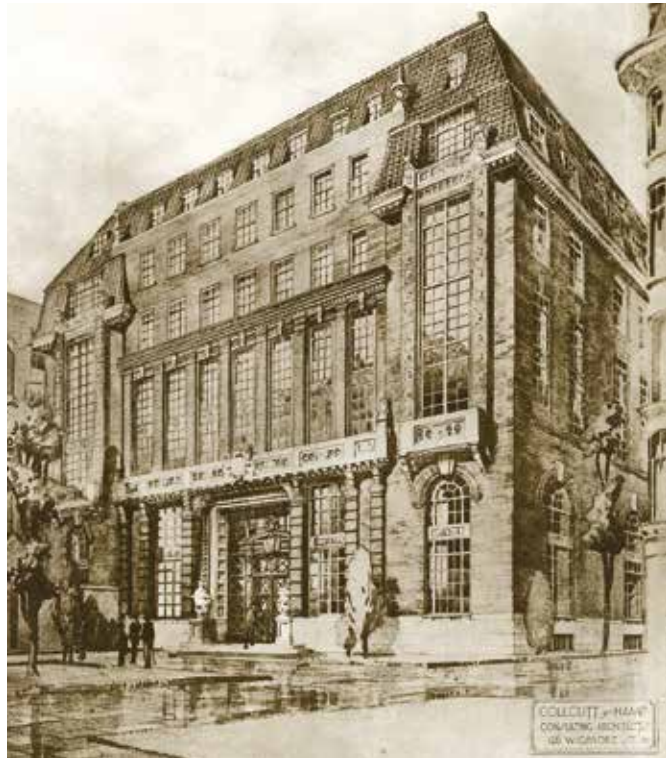
Stanley Hamp's elevational drawing of Haddon House used in the original letting brochure, which described the elevation as 'of Spanish Renaissance design, executed in red brick, with stone embellishments and red-tiled roof'.
