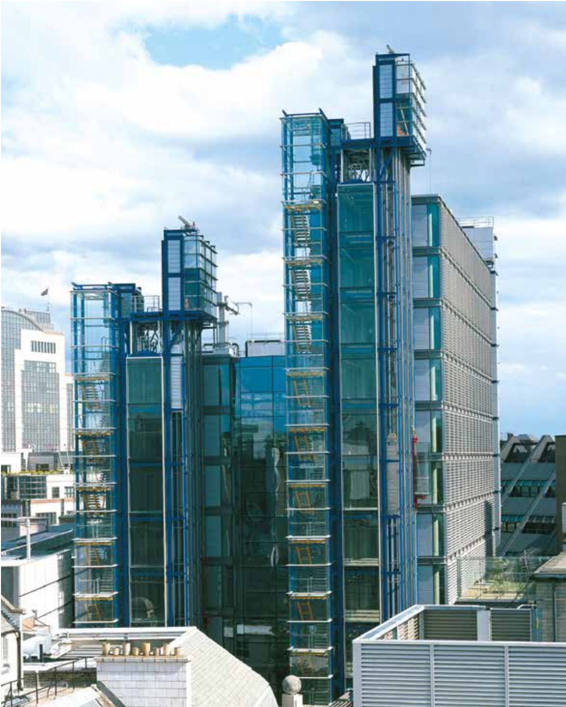
A view across the roof tops of Fenchurch Street to the Rogers building. The motor rooms of the wall-climbing lifts give a distinctive shape to the top of the two front towers.
