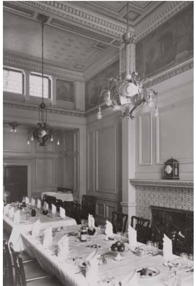
The Classing Room was originally the Luncheon Room. Note the clerestory windows.
