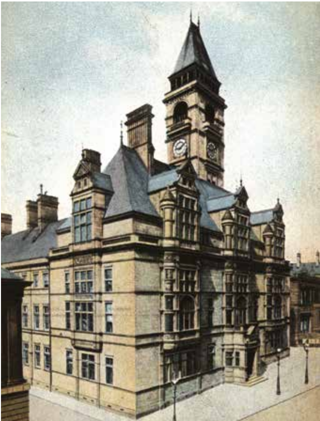
Collcutt won the competition to design Wakefield Town Hall in 1877 and the building was officially opened in 1880. He also designed the interior of which much survives, including the Council Chamber containing rich relief decorations, carved fireplaces and fine woodwork.
