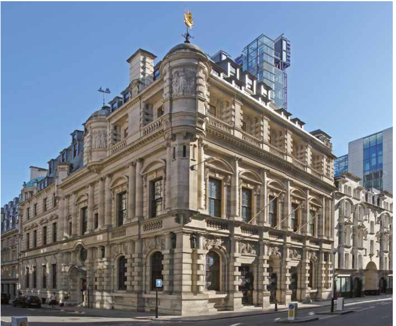
Collcutt's building stands solidly on the corner of Fenchurch Street and Lloyd's Avenue. The Rogers building appears just above it. Coronation House is on the left and the double height archway in Nos. 68-70 Fenchurch Street, which is now the main entrance to the complex, can be seen on the right. These buildings are described on page 27.
