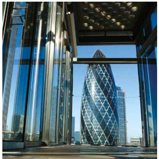
The front lifts and stairs also provide wide views across London for those with no fear of heights. Concrete flooring with glass 'portholes' is used in the landings. This flooring also forms the ceiling to the landing areas, as seen here.
