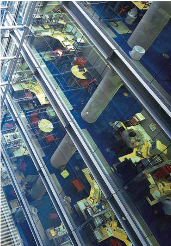
The atria bring light into the building and mean that more employees benefit from direct daylight at their desks.
