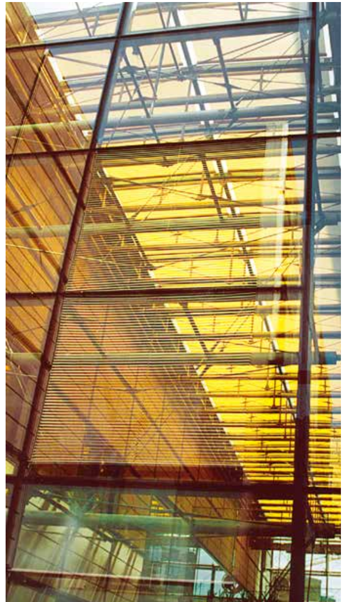
Bright yellow blinds flood the atria and offices with colour when the sun activates the environmental control system.
