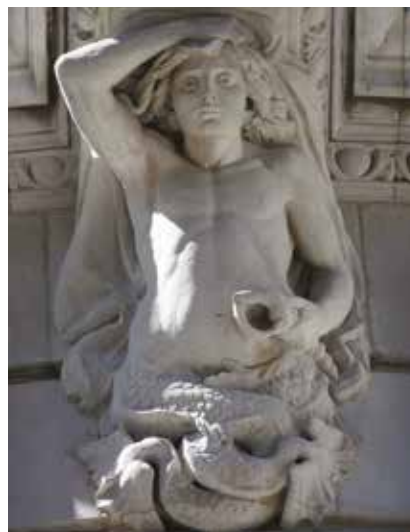
One of Taylerson's figures, a merman, supports a second floor column on the round tower between the second and third palaces.
