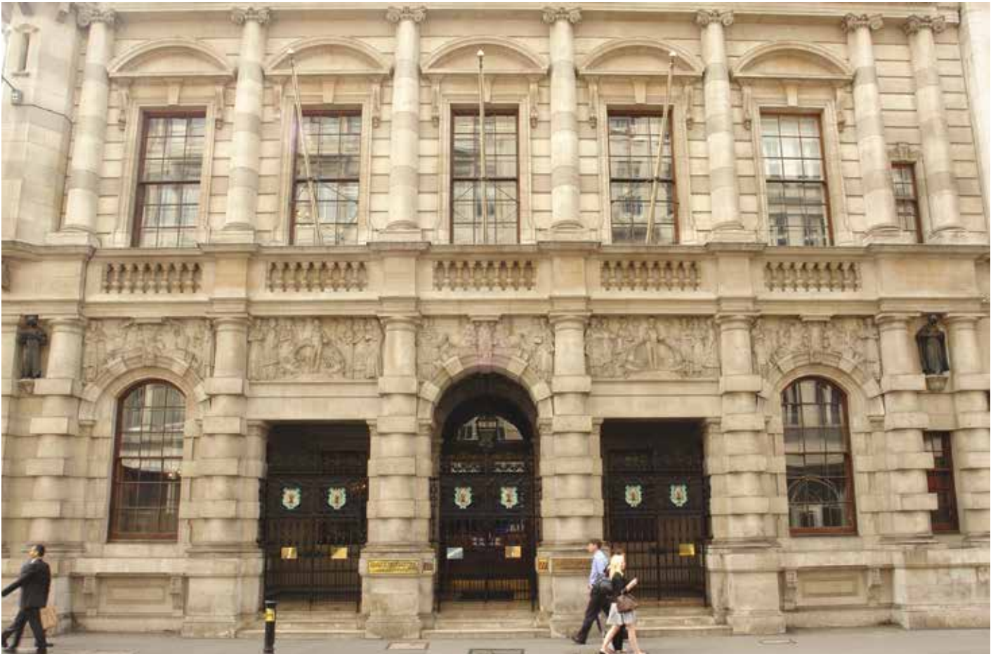
The Fenchurch Street façade is richly decorated with the tableau by George Frampton; detail of the scene below shows Mercury flanked by ships and maidens. The wrought iron entrance gates are now usually kept shut as the main entrance to No. 71 is through Nos. 68-70 Fenchurch Street and the Rogers building.
